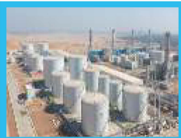
Assiut Add-On Power Plant 500 MW PCESCO / EGYPT
