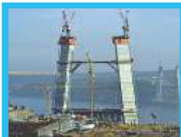
Yavuz Sultan Selim Bridge ISTANBUL / TURKEY
