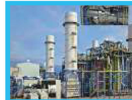
New Capital Power Plant 4800 MW PCESCO / EGYPT
