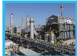
Azmeco Methanol Plant BAKU / AZERBAIJAN
